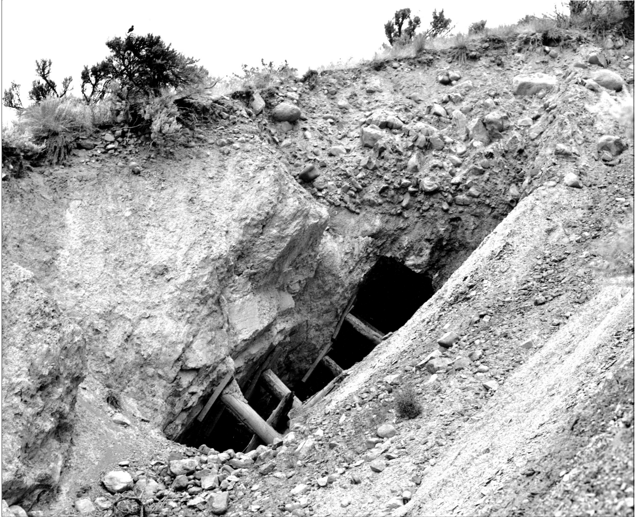
Figure 73. Upper adit, Consolidated Mine, June 25, 1966. Photo by Peter Oberlindacher, BLM.
